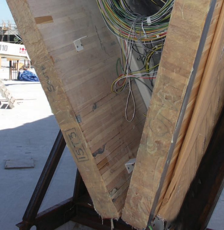
A composite twin glulam beam arch section cavity complete with services
