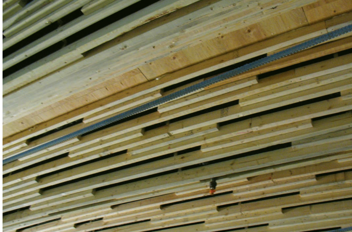
Panel Vees – underside
