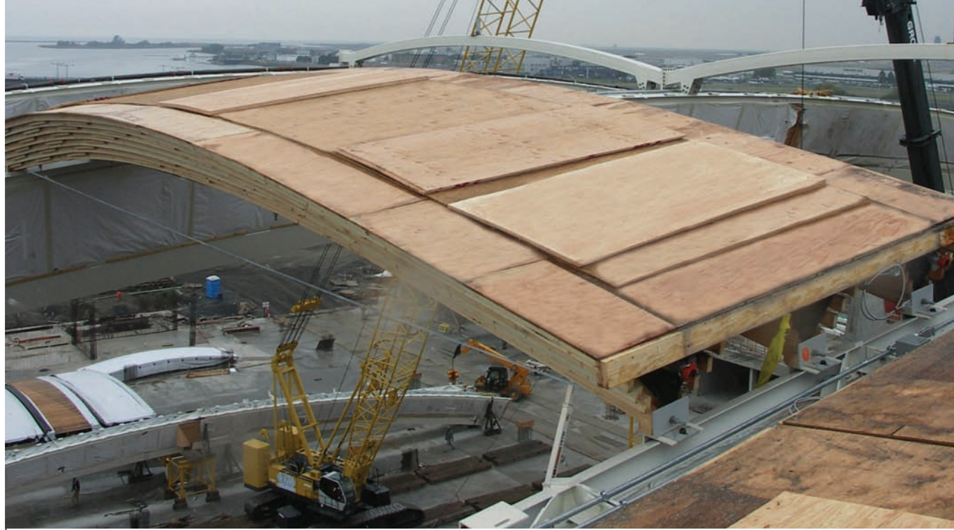
WoodWave panel bolted in place to a pair of glulam arches
