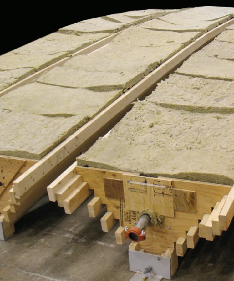
Panel Vees loaded with fibrous insulation
