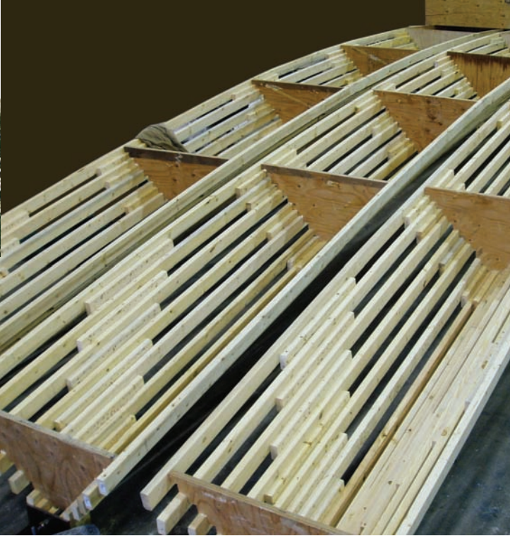
Panel Vees - staged prior to assembly
