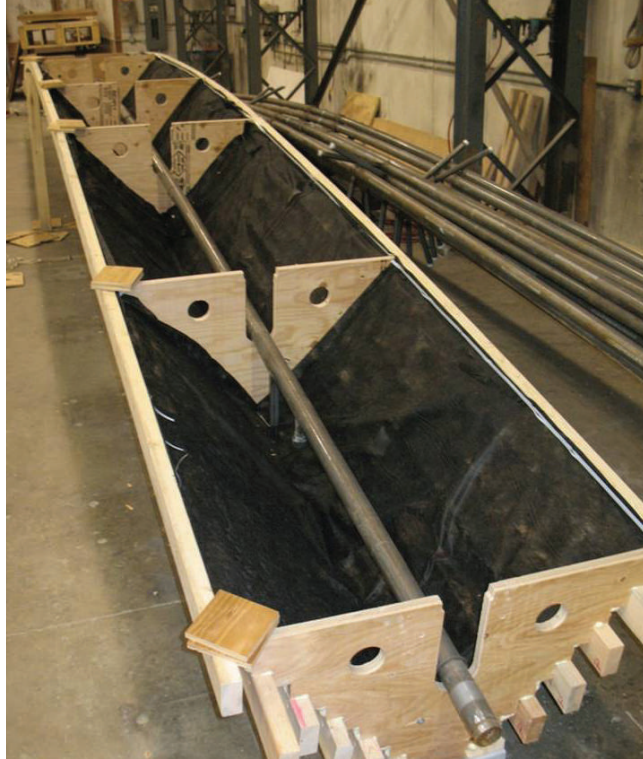
Panel Vee with sprinkler line positioned, lined with fabric and plywood gussets drilled for services
