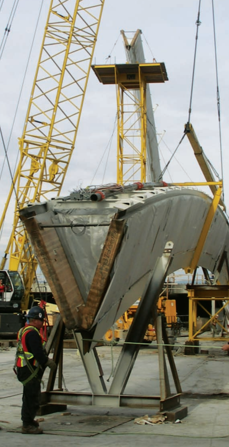
Ventilation system main duct fabricated within the glulam arches cavity
