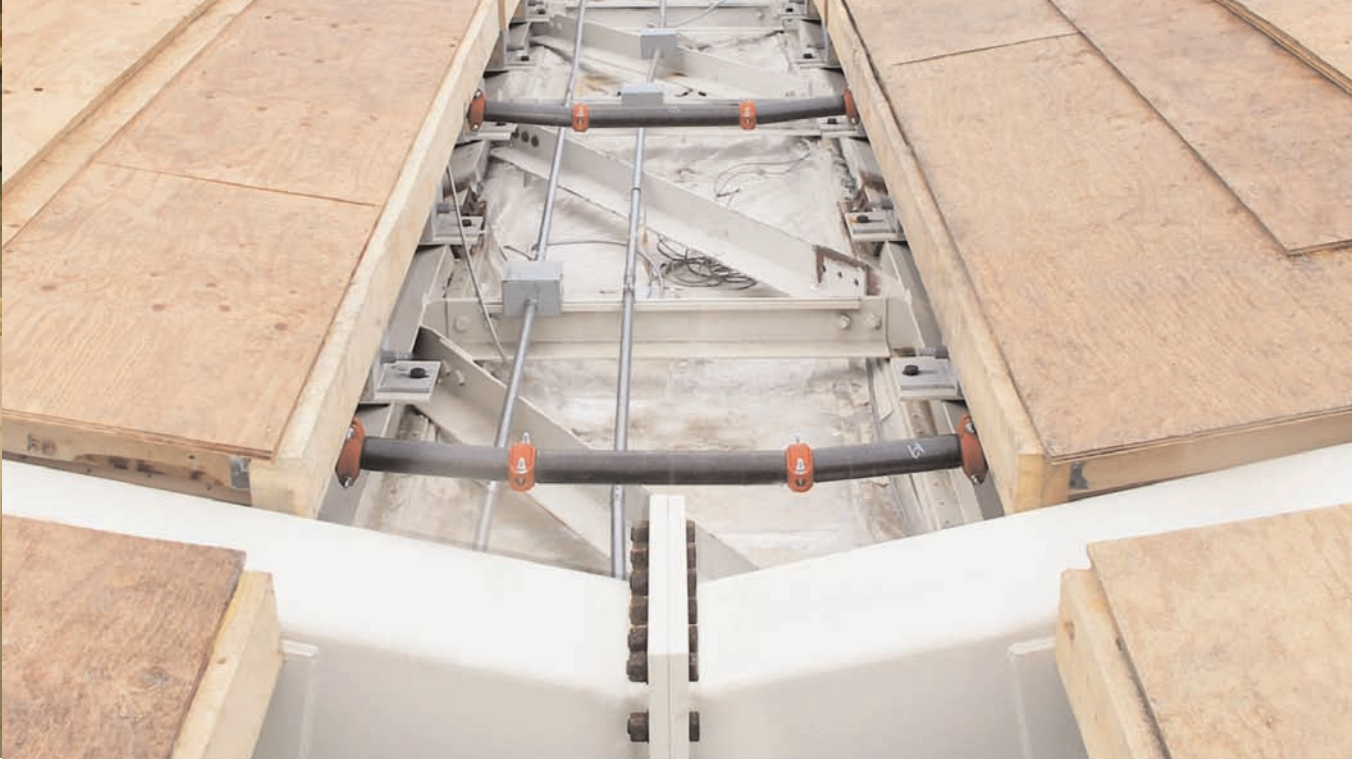
Top down roof view of an arch prior to sheathing; sprinkler system main lines, electrical conduits, ventilation system ducting, strut connection detail, WoodWave panel to arch connection detail, glulam arch steel forming and bracing elements
