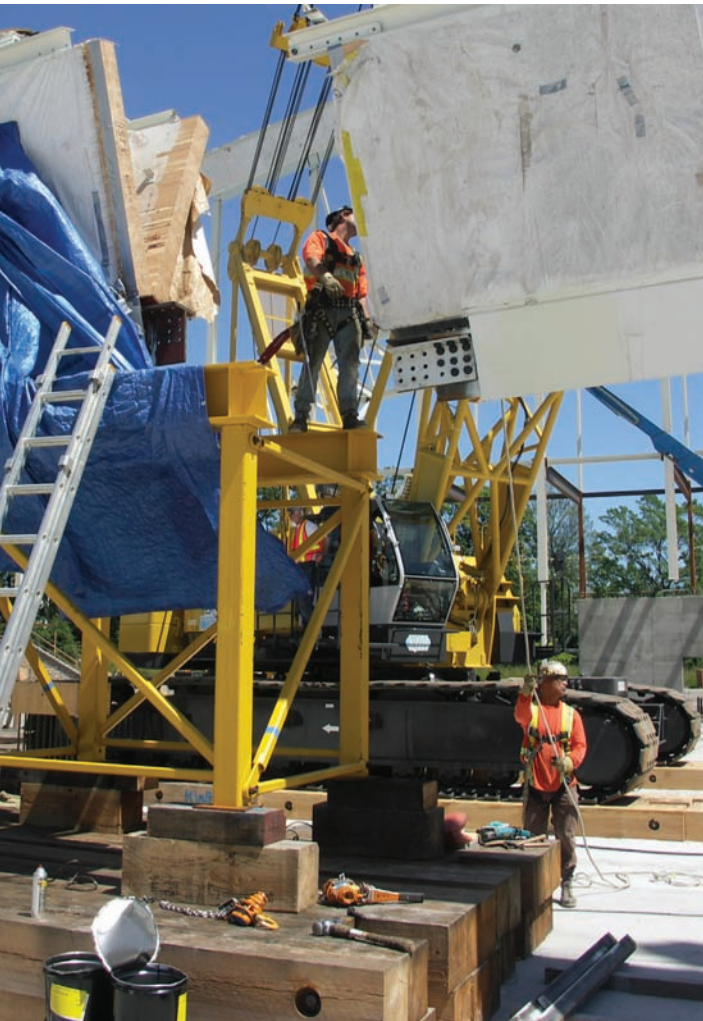
Staging of glulam arch sections on the site slab prior to the final connection of the two center span sections
