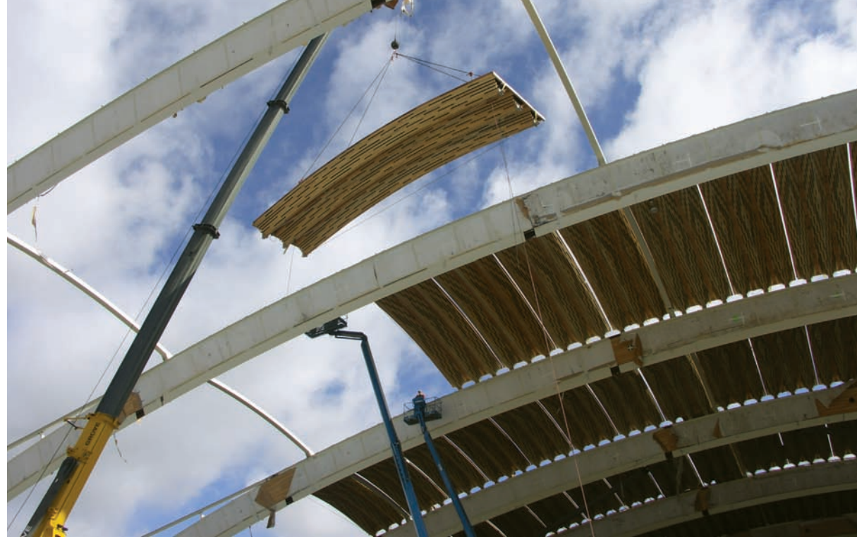
Placing a WoodWave panel
