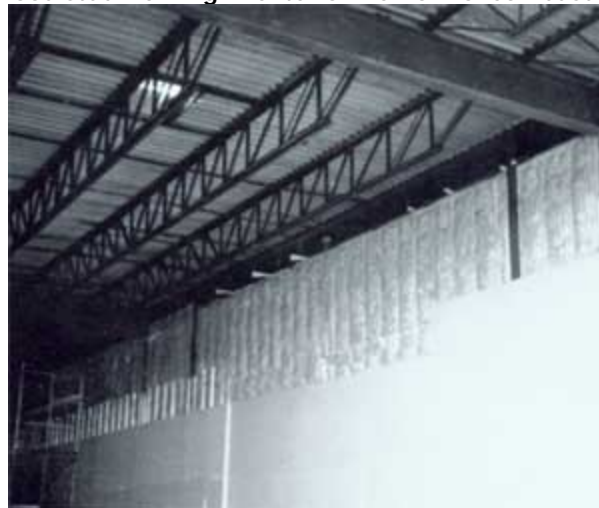
Figure 2: Wood stud framing in exterior wall of noncombustible building
