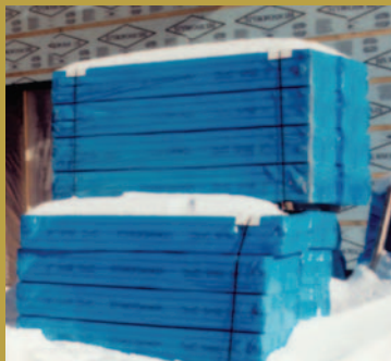
Figure 9: Well protected bundles
